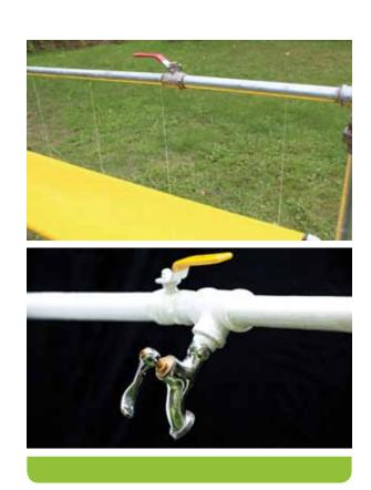
To minimize water usage, a faucet is provided on the side of the punch pipe to allow individual handwashing without assistance.
