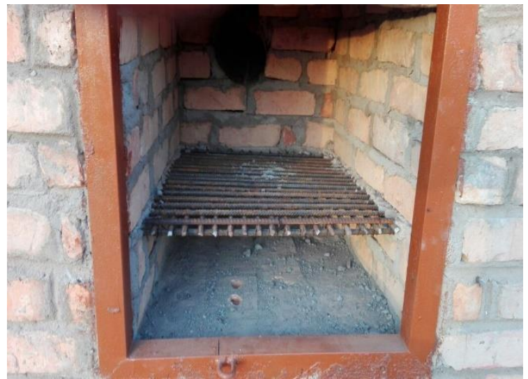
Fig. 2: Used pad chamber/ incinerator in full (left picture), and inside of the pad chamber /incinerator (top picture)
