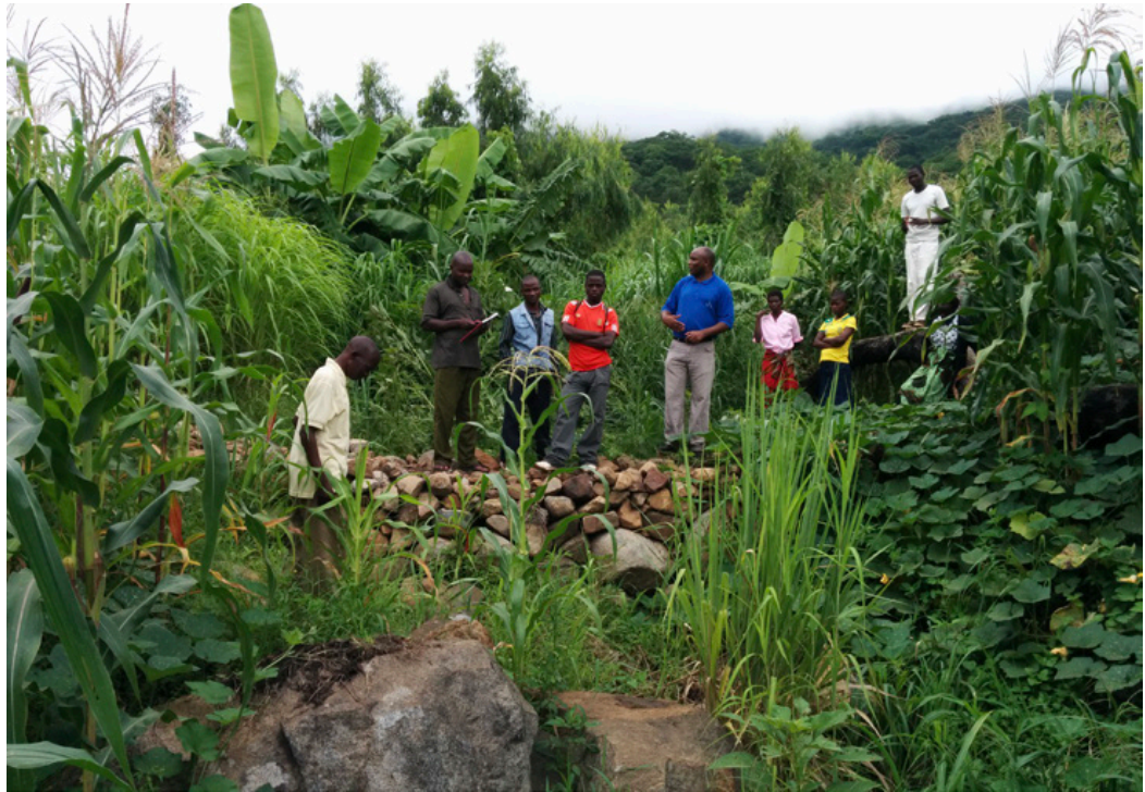
Members of the Watershed Committee standing on a large (about 12-m) check dam, which has reclaimed a barren gully, Lingoni. Photo by Chris Reichert for CRS.
