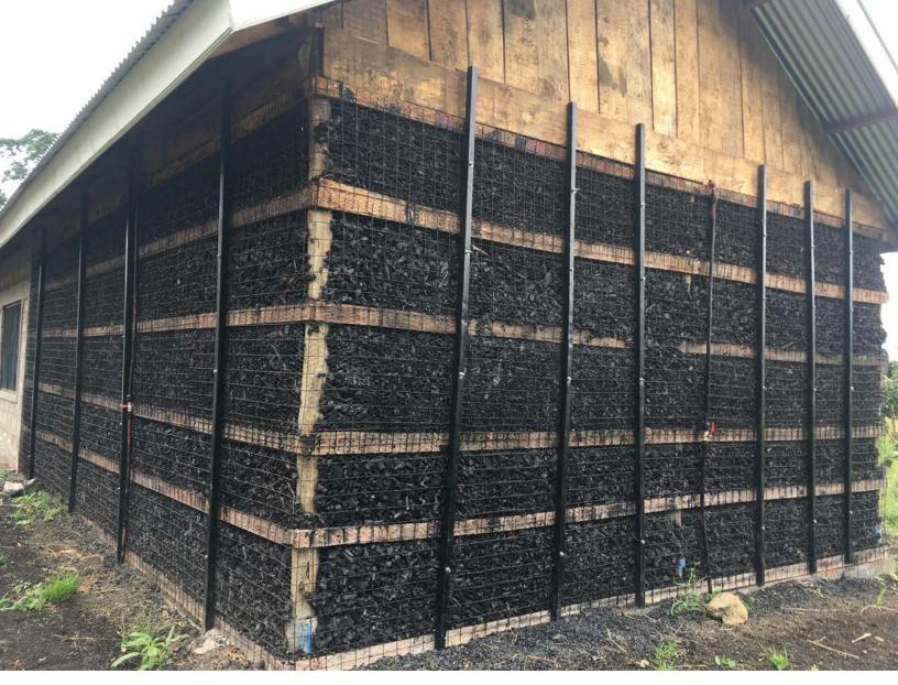
Cold storage room in Tanzania using charcoal-filled siding. The appropriate technology creates conditions for cold storage without the use of fossil fuels.
