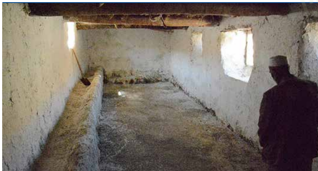
Figure 1: An improved stable with ventilation, light, well-drained floor, raised feed trough and limewashed walls.
