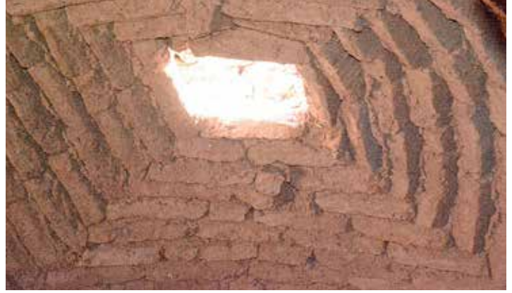
Figure 3: A farmer's improved roof ventilation
