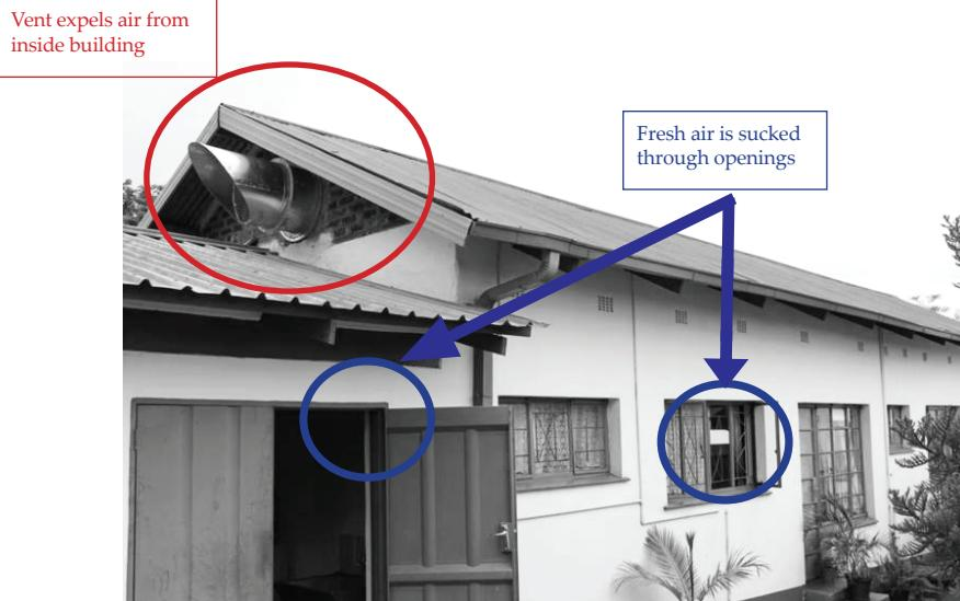
All of these low cost, low maintenance systems are suitable for installation in both permanent and semi-permanent constructions. However, they did present some challenges, including high noise levels created by ducts (solved by installing sound reducers), extractor fans not working correctly, and in some cases, weak public electric systems with insufficient amperage to power the ventilation systems.
