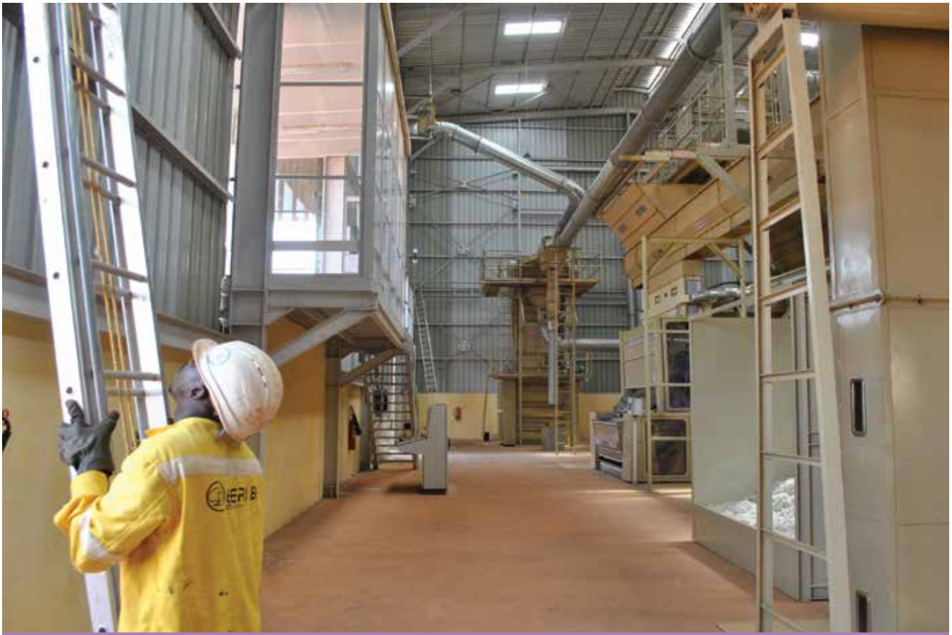
Ginning machinery inside the newly constructed organic-priority gin. Photo by CRS
