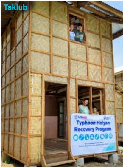
Above: The Taklub—from the Waray Waray word *Tarakluban*, Tacloban City’s old name—was developed during this response and is a two-story model with a kitchen, adapted from the Pablo elevated style. *Taklub* is fishing gear used by fishermen and, in the local dialect, means “cover”. Left: The Bohol (named after the earthquake which hit the island of Bohol in 2013) has a 0.6-meter base made from concrete hollow blocks and walls made from *amakan*.
