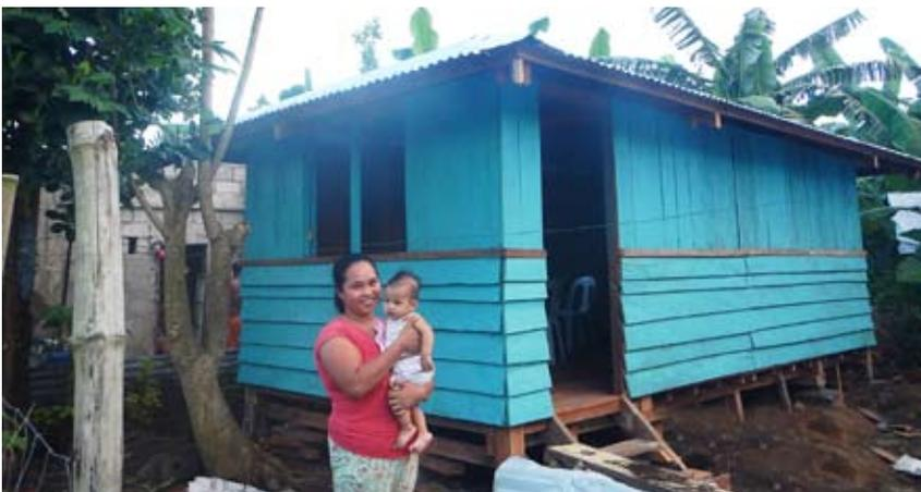
CRS piloted the use of coco lumber walling to replace the *amakan* bamboo walling in response to community feedback.
