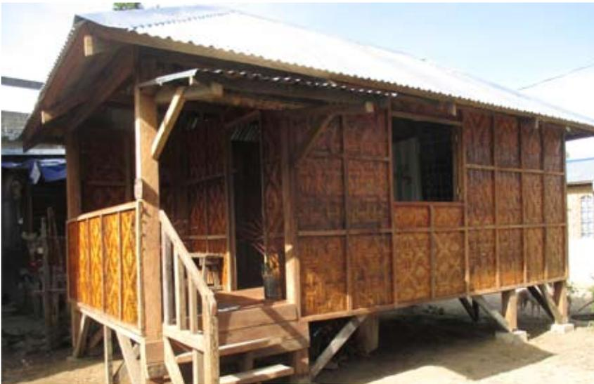
In December 2014, CRS changed the roof on the Pablo direct-build shelters from a gabled roof to a hipped roof.
