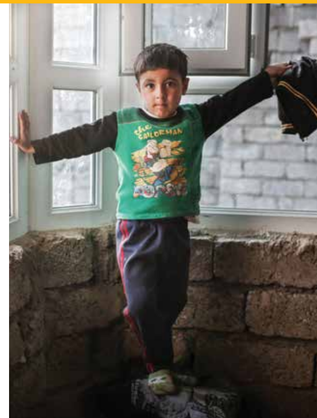
A newly installed double-glazed window keeps out cold winter air in the house that Raybas Dorbo, 4, a displaced Yazidi from Sinjar, shares with his family. The partially constructed house near Dohuk was renovated by CRS partner Caritas. Photo courtesy of Sam Tarling/Caritas
