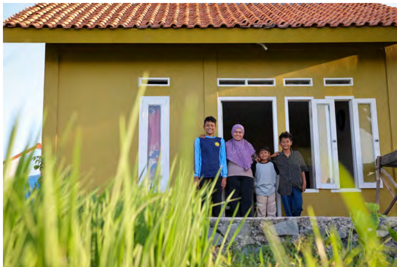
Tisah and her family in their newly constructed district home after it was nearly destroyed by heavy storms in Indonesia's Tangarang district. Photo by Benny Manser/CRS
