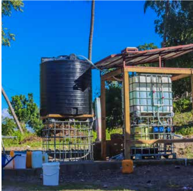
A water treatment system installed by partner Water Mission International in Boumier, Les Cayes. Photo by Franklin Gentillon/CRS
