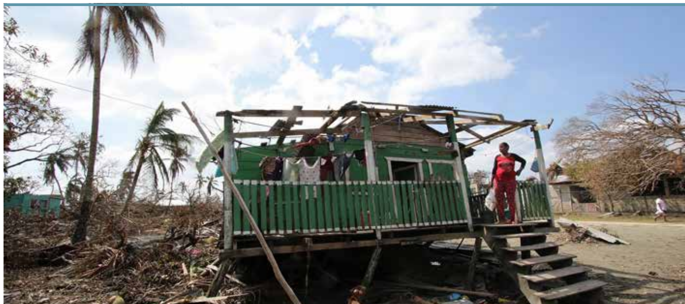
Destruction caused by Hurricane Eta in Nicaragua in November 2020. EMPOWER supported Caritas Nicaragua in a rapid emergency shelter and WASH response to the Category 4 hurricane. Photo by Katlyn Holland/CRS
