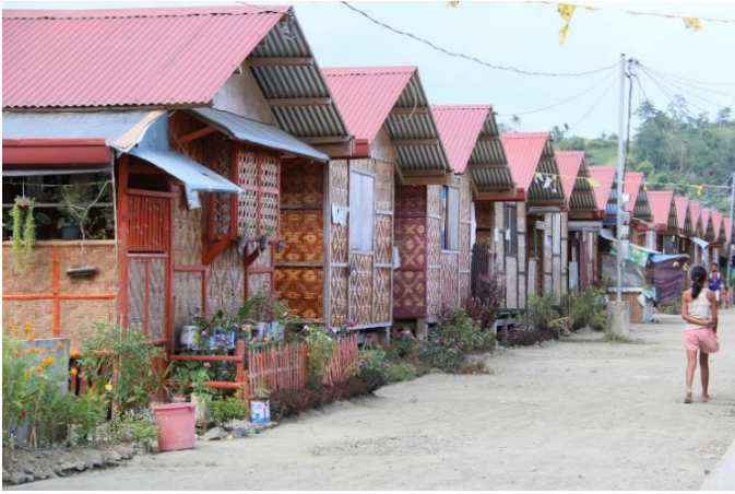
After Super Typhoon Haiyan slammed into the Philippines in 2013, CRS supported the reconstruction of 20,000 homes. In December 2014, the homes withstood a typhoon and tropical storm with minimal damage. Photo by Kim Pozniak/CRS
