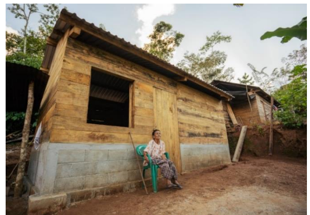
CRS helped Mercedes rebuild her home in Guatemala after it was destroyed by hurricanes Eta and Iota. The home was built using low-cost hurricane resilient techniques, including concrete blocks and boards for walls and a concrete floor. Photo by Dinorah Lorenzana/CRS
