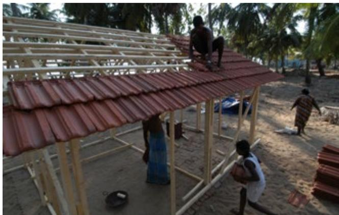
Workers labor to roof a CRS/Caritas provided temporary shelter in Navalady, one of 86 such homes provided by CRS/Caritas in the community, which was nearly wiped out by the tsunami. In all, the roof consists of 400 clay tiles, each costing about .14 cents, which help to keep the insides of the homes cool in temperatures exceeding 100°F (38°C) in the hot months.
