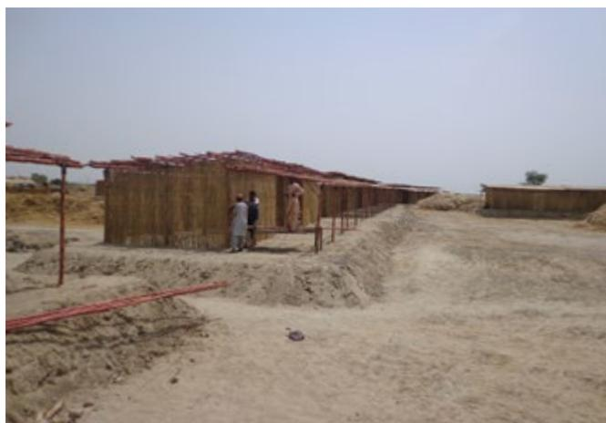
Building shelters on a raised plinth is one of the most effective ways of reducing damage to shelters during flooding. Drainage ditches were dug with stone or earth curbs dug around the perimeter of shelter to divert rainwater away from the house. A small number of non-beneficiary households replicated the technique when building their own houses.
