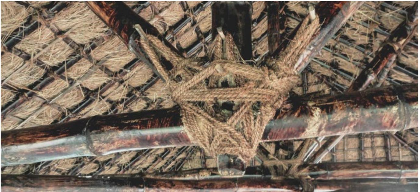
Beams and wall joints use locally produced natural fibres which can be easily repaired or replaced and do not compromise the strength of the bamboo poles
