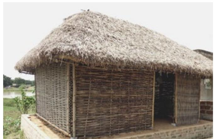
The woven split bamboo mesh walls are then mud plastered inside and outside, once the hipped roof is completed
