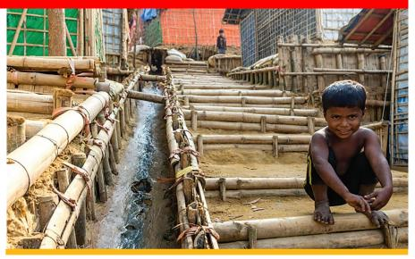
Through a CRS cash-for-work activity, Rohingya refugees used local materials to build structures such as drainage and terraces to mitigate erosion and flooding in the refugee settlement. *Photo by Christopher Reichert/CRS*
