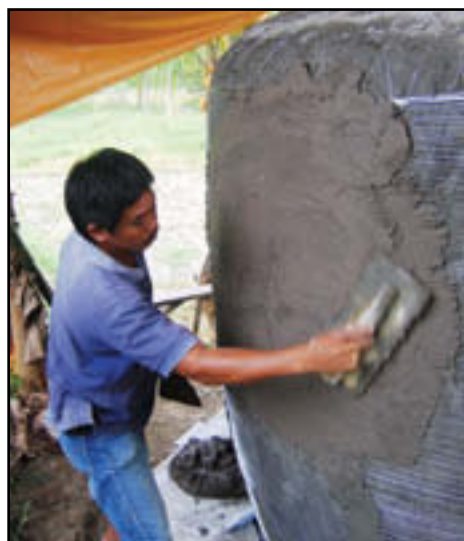
Fig. 67: Applying the final layer
