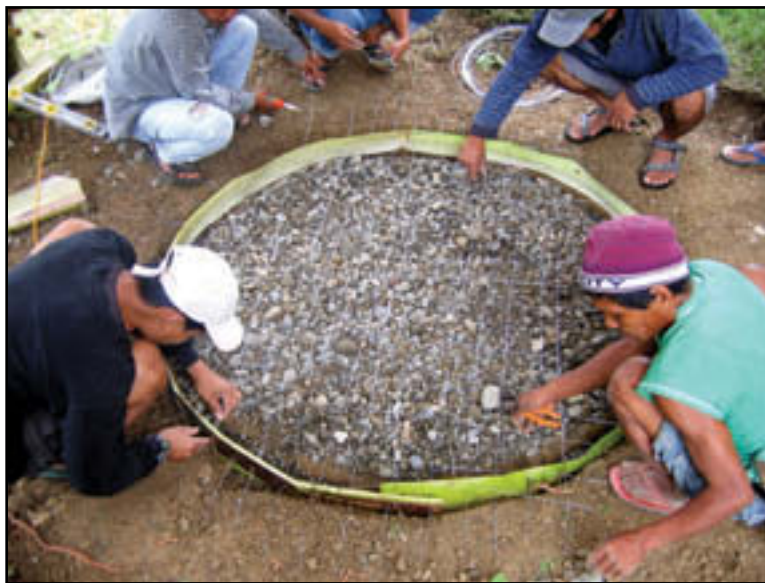
Fig. 51: Adding base reinforcement
