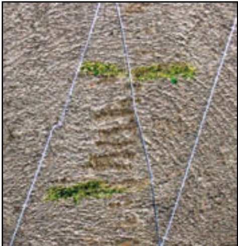
Fig. 65: Marking horizontal wire placement
