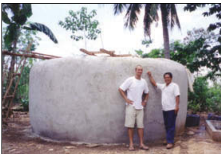
Fig. 12: The Wire-Reinforced Jar — a 30,000 liter tank in Camotes, Cebu, Philippines
