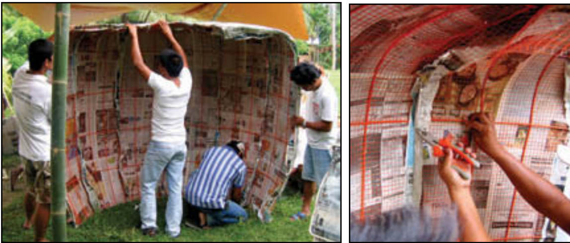
Figs. 54-55: Assembling the form
