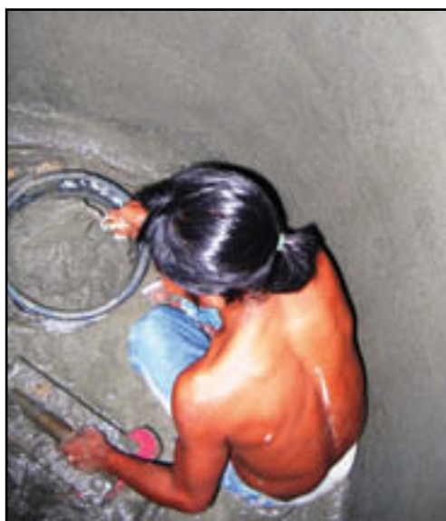
Fig. 71: Plastering the inside of the tank
