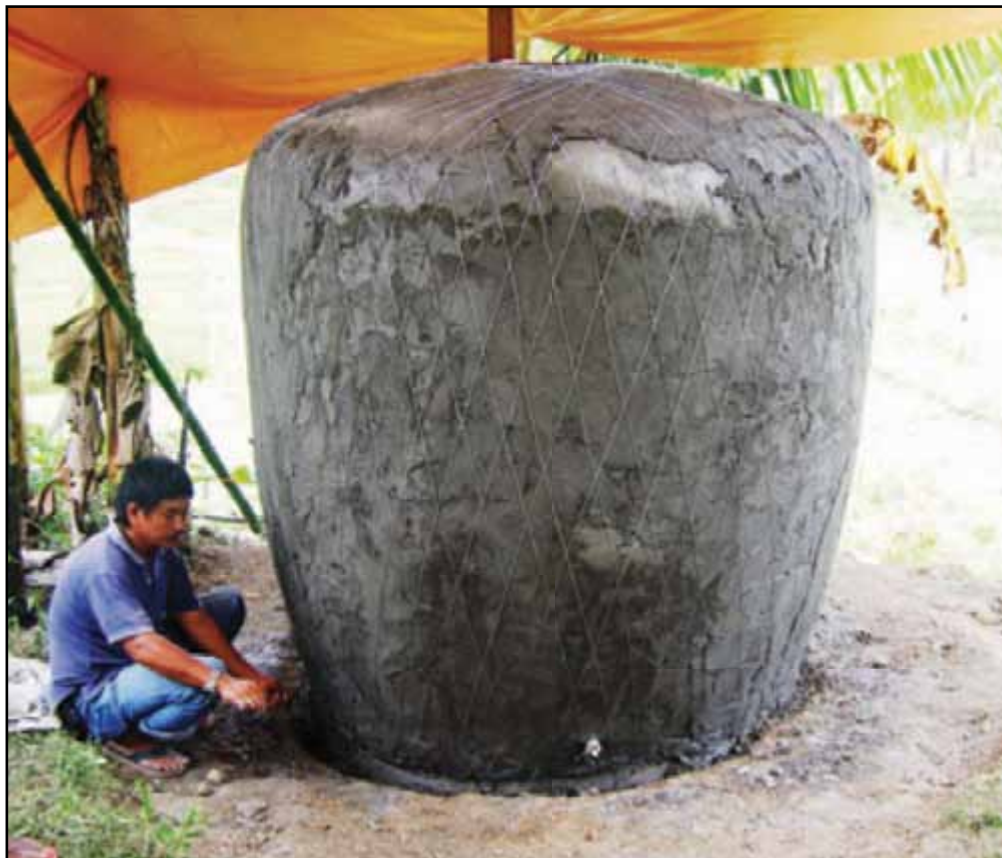
Fig. 63: Completed vertical wire reinforcement
