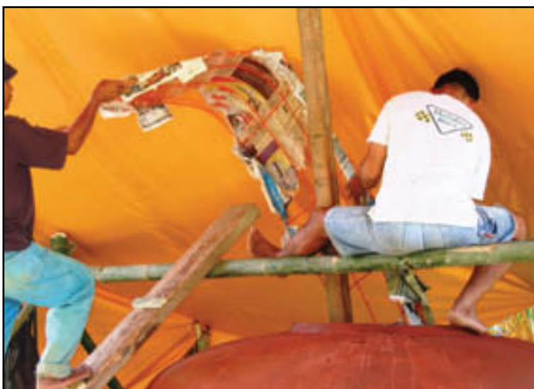
Fig. 70: Removing the form
