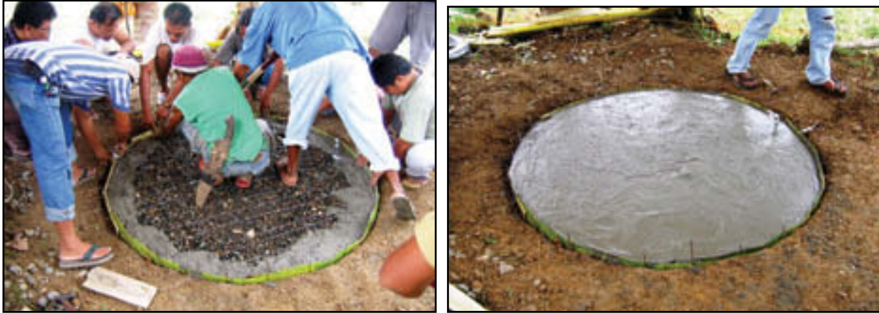
Figs. 52-53: Pouring cement and The completed base
