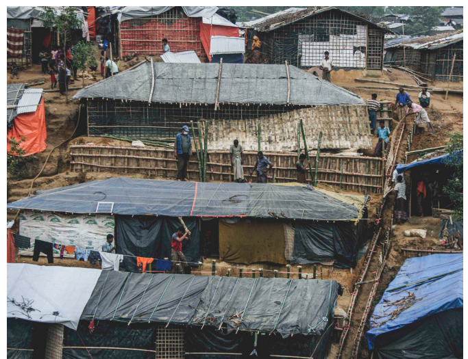
The community working on installing drainage and retaining walls.
