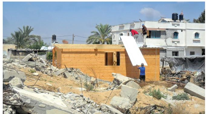
Contractor staff placing CGI roofing on the shelter.
