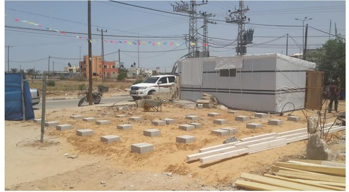
Laying the foundation and ground beams for the transitional shelter.
