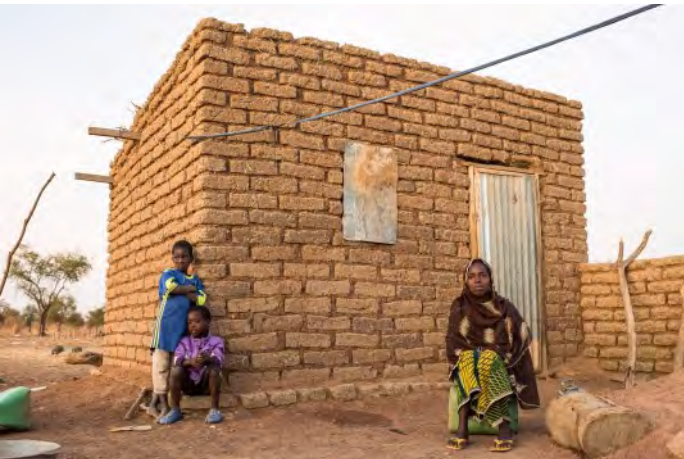
Shelter maintained via SILC support, Goudrin village, Toungouri commune, 2017.
