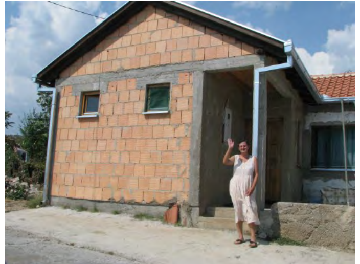
Home repairs for returnees in Kozice, 2008.
