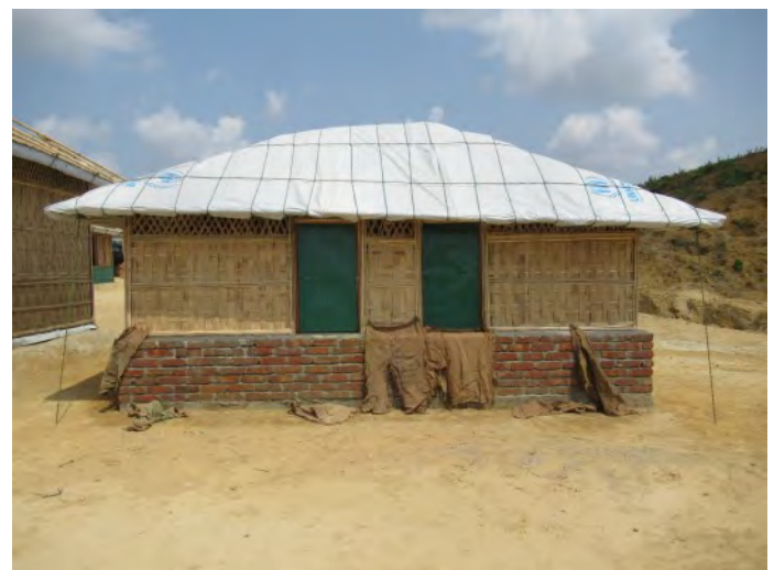
Midterm shelters - Kutupalong Expansion Site, 2018
