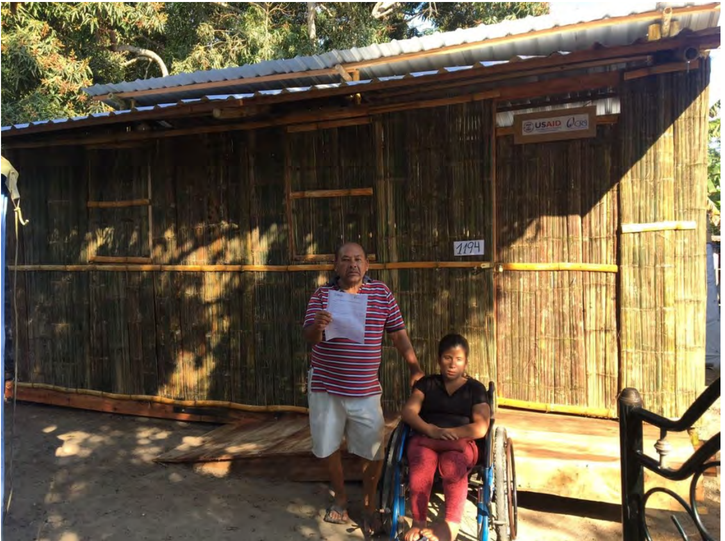
Transitional shelter built with bamboo and timber, Bigua, Manabí province.
