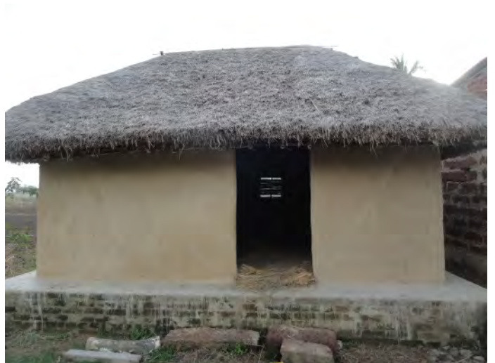
Permanent shelter, elevated to reduce risks of flooding, 2017.
