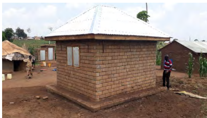
12m² shelter completed. 2019.
