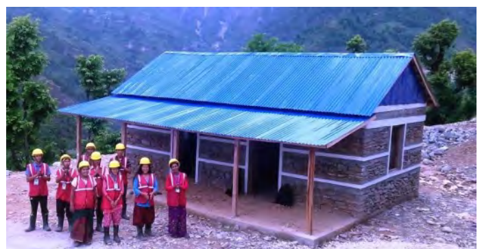
Complete demonstration house in Arupukhari, 2017.
