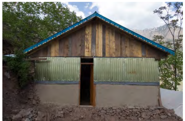
Transitional shelter using mixed materials, 2006.
