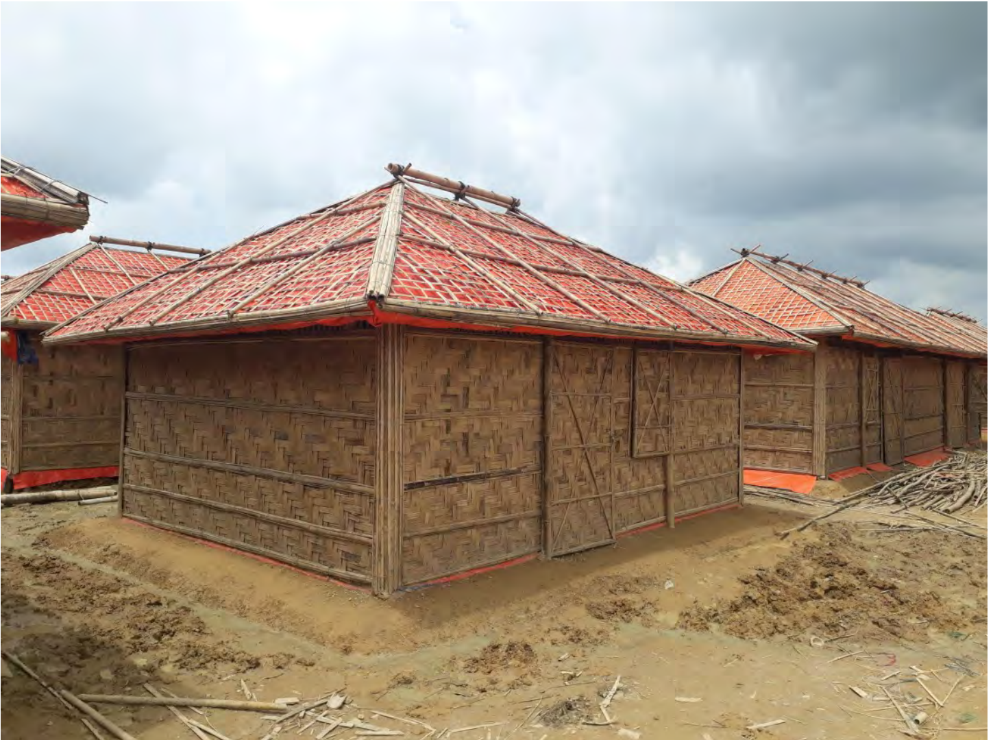
Midterm shelters - Kutupalong Expansion Site, 2018
