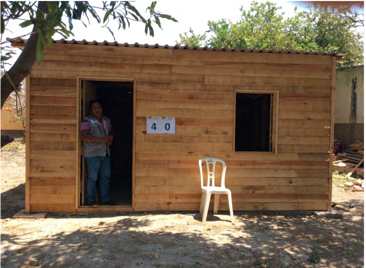
Transitional shelter using continuous concrete foundations and reinforced wooden structure, 2018.
