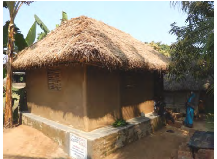
Shelter using improved techniques such as elevated foundation and weather-resistant plastering, 2015.
