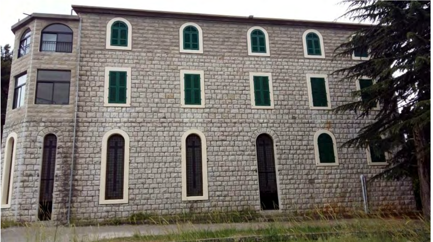
Rehabilitated Bhersaf Shelter hosting migrants and managed by Caritas Lebanon Migrant Center. The works included repairs on the heating and sanitation system, the roof weatherproofing, removal of wall mold, maintenance of doors and windows and general painting, 2016.
