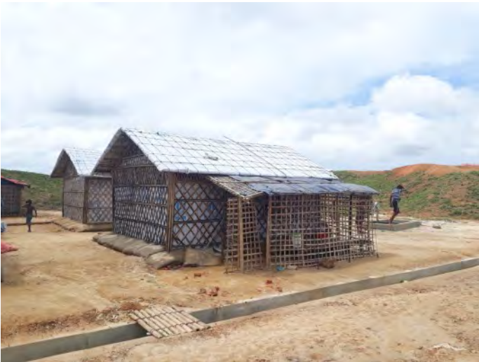
Transitional shelters - Kutupalong Expansion Site, 2018
