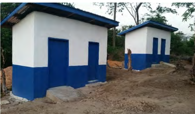
School latrines in Niene Chiefdom, 2016.
