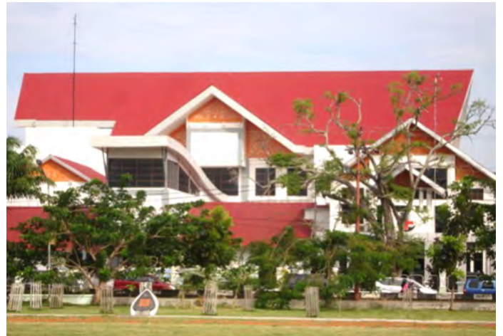
78 bed capacity Maternity Hospital at Banda Aceh, Indonesia 2009.
