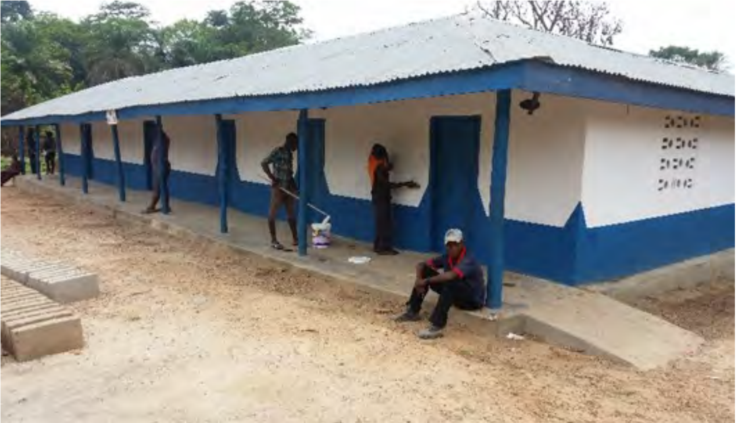
Construction and rehabilitation of classrooms, in Niene Chiefdom, 2016.
