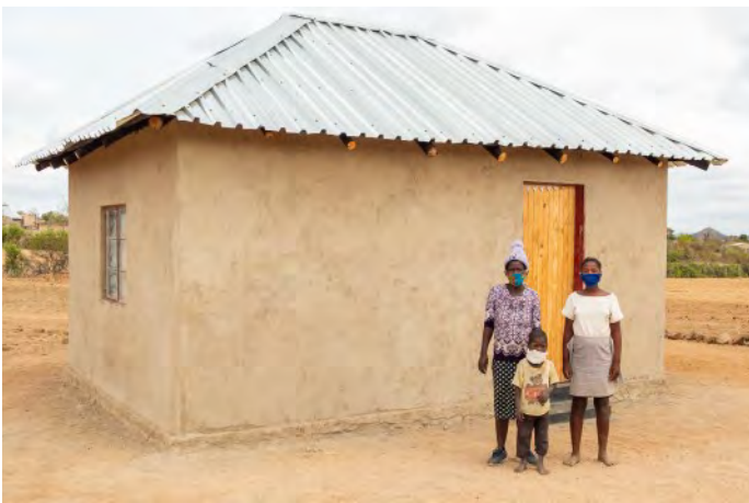
Tamary Tivakudze and her family benefitted from a two-bedroom shelter in ward 27, Buhera South. Their shelter had rooms of different sizes.
