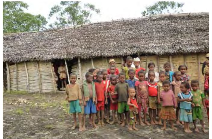
School facility assisted with minor improvements during the response to Cyclone Ava
