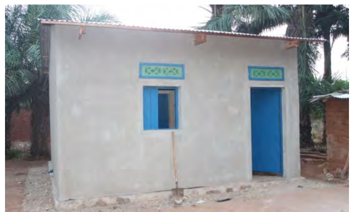
One bedroom, durable shelter with external plaster, 2019.
