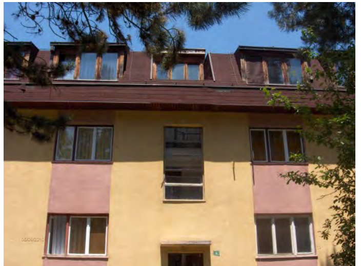
Housing building retrofit, Gorazde, 2011
