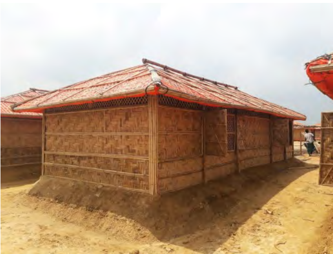
Midterm shelters - Kutupalong Expansion Site, 2018
