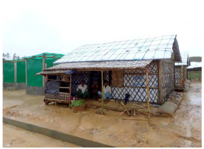
Transitional shelters - Kutupalong Expansion Site, 2018
