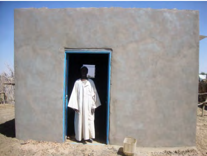
Permanent shelter made of mud bricks, West Darfur, 2014.
