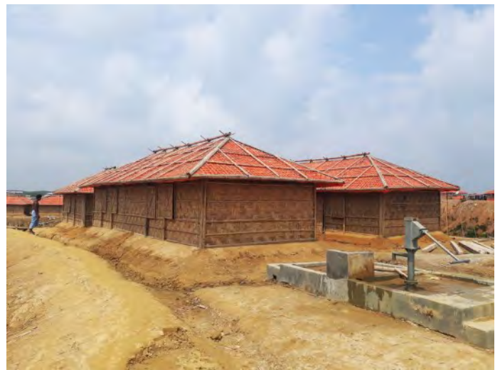
Midterm shelters - Kutupalong Expansion Site, 2018
