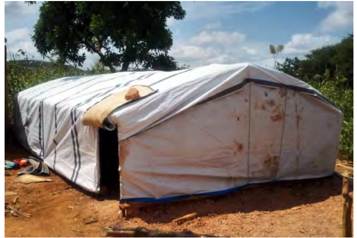
Emergency shelters are built using a combination of in-kind and cash assistance, Kaya, 2020.
