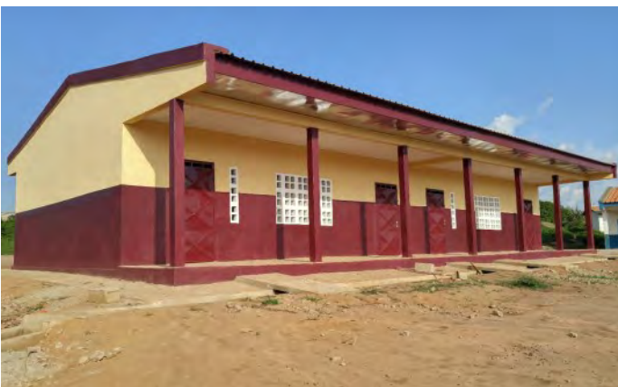
New classrooms in Kadey Department, 2016.
