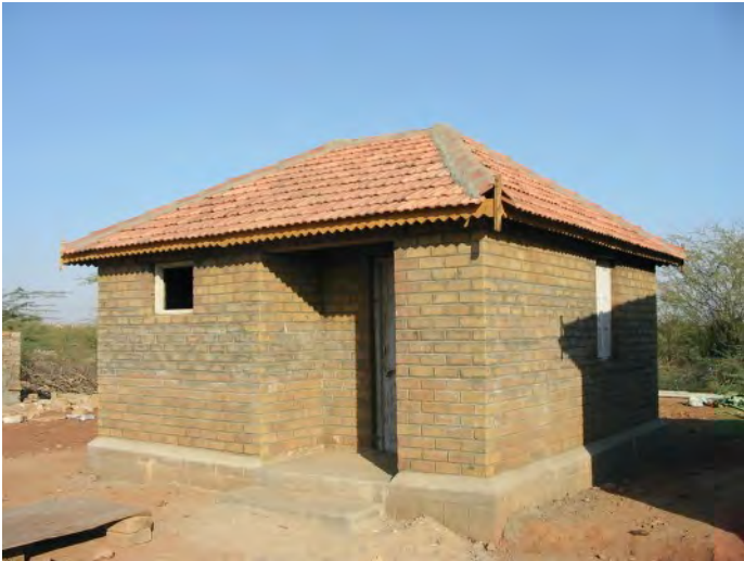
Permanent disaster resilient shelter featuring roof tiles, Gujarat, 2004.
