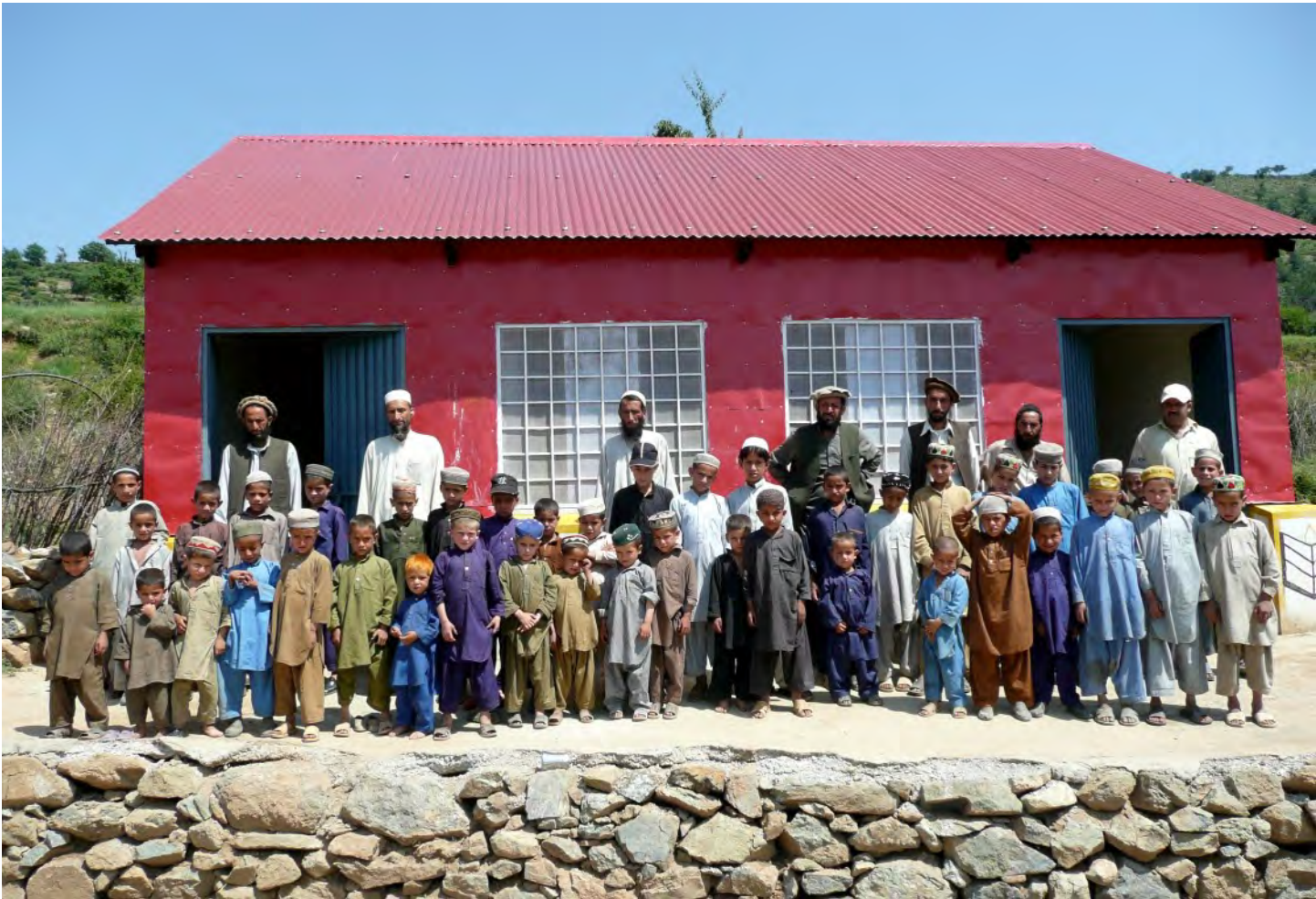
Primary school rehabilitated in Bar Gabar Village, 2007.
