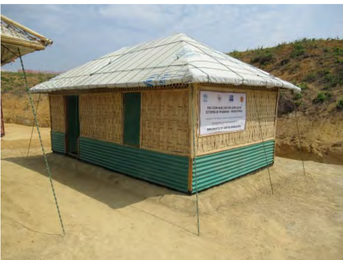
Midterm shelters - Kutupalong Expansion Site, 2018
