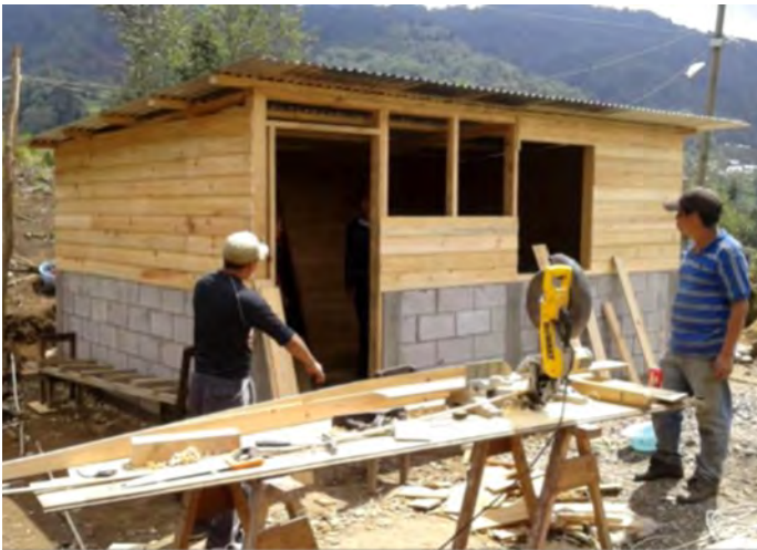
Construction of a permanent, post-earthquake shelter in San Marcos, Guatemala, 2014.
