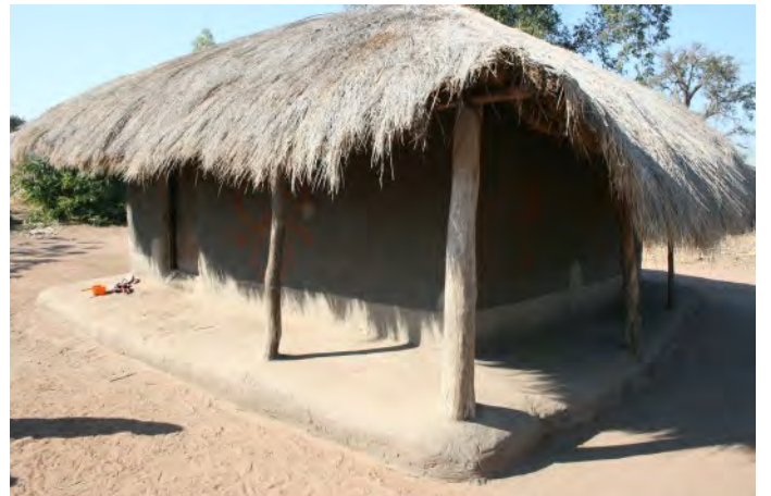
Shelter built with traditional techniques, 2015.
