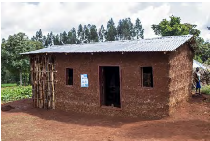
Permanent shelter built where a temporary shelter was placed before, with support from DFID, in Gelcha kebele, Gedeb woreda, Gedeo zone, 2019.
