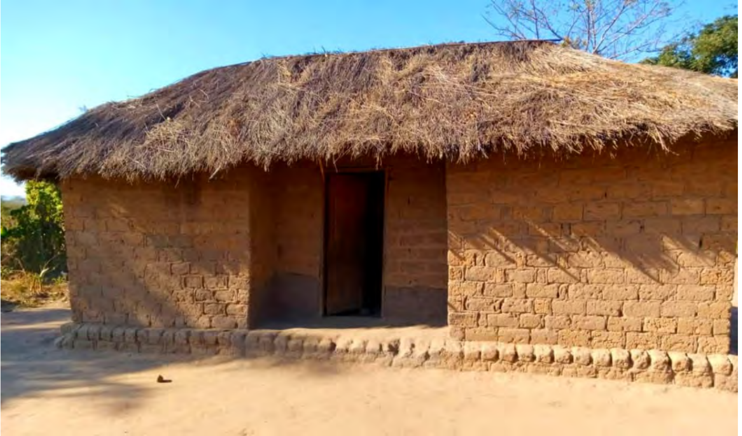
In the remote rural areas of DRC, families rebuild permanent shelters using adobe bricks and thatch roofs. 2015.
