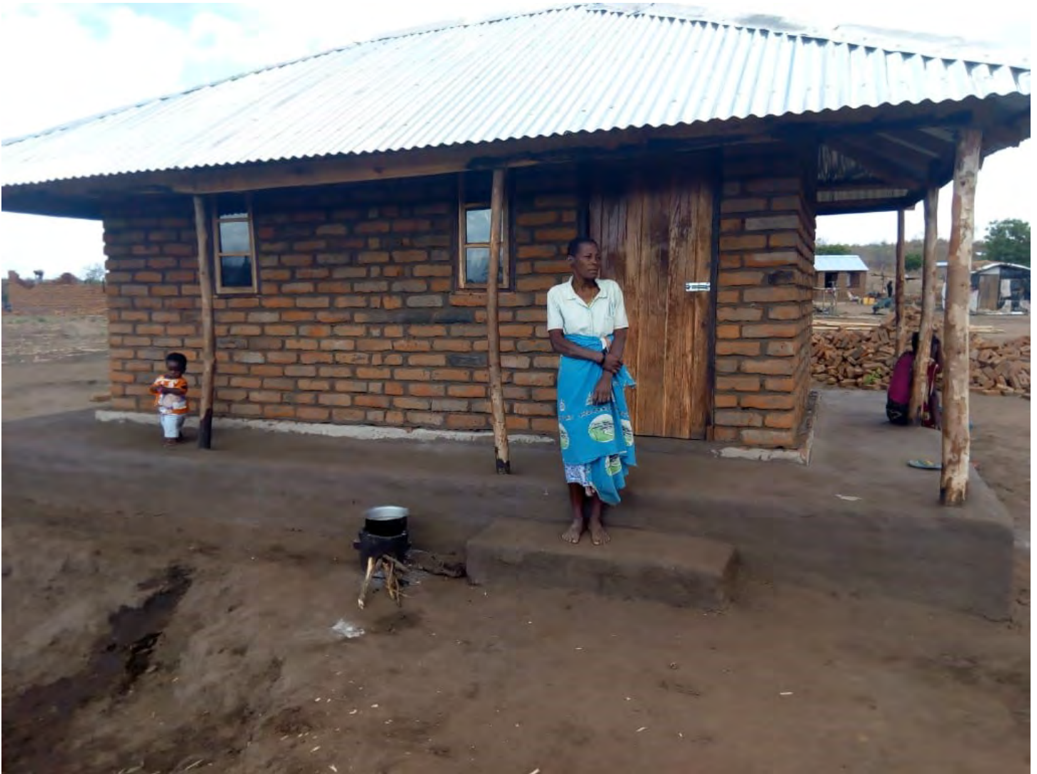
Shelter built using improved, local techniques in Mwalija village, 2019.
