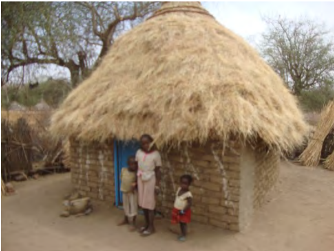
Transitional shelter made of mud bricks, West Darfur, 2014.
