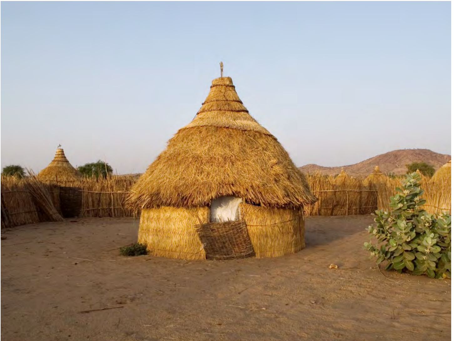
Gutia round mud and thatch shelter built with emergency assistance, West Darfur, 2005.
