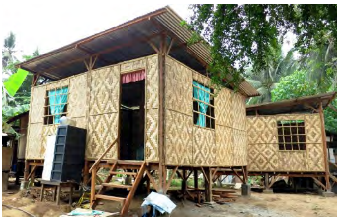
Transitional shelters built by CRS after flash floods, Cagayan de Oro, 2011-2012.
