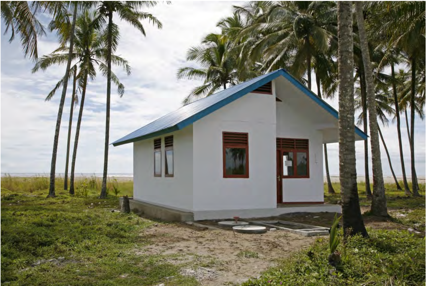
Permanent house, built with internal sanitation facilities, Meulaboh, Aceh, 2007.
