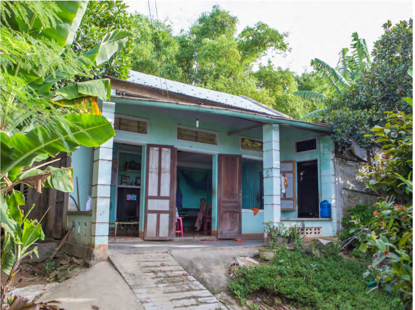
Le Thi Phuoc's home, retrofitted and renovated replacing the roof to withstand strong storms.
