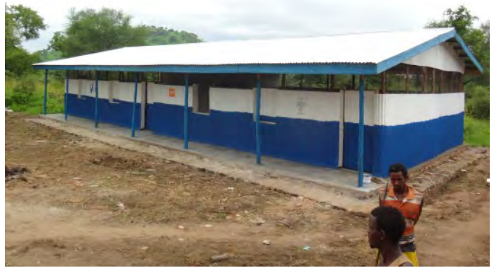
Two classrooms blocks constructed by CRS at Kule
