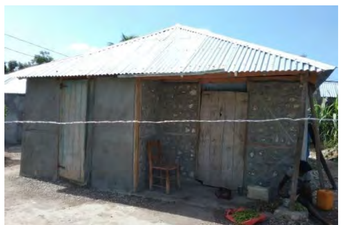
Reconstructed transitional shelter for a family of nine, 2017.
