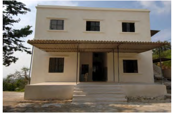
Small building rehabilitated and then used as a youth center and social club, Aktanite, 2007.
