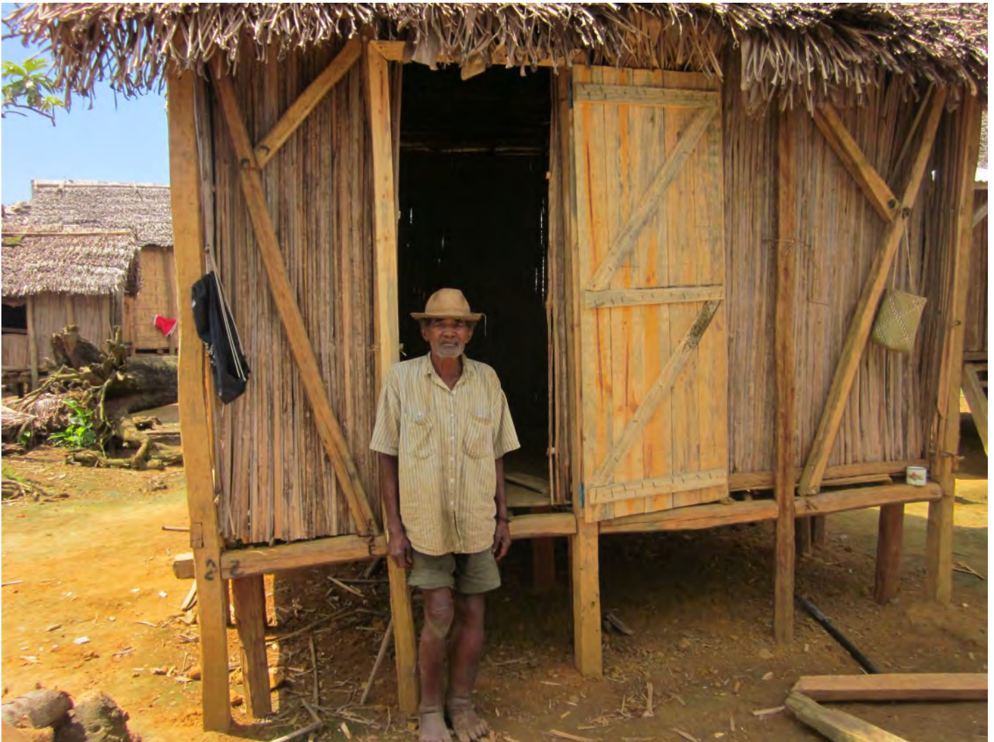
Completed shelter unit, elevated and braced against high winds.
