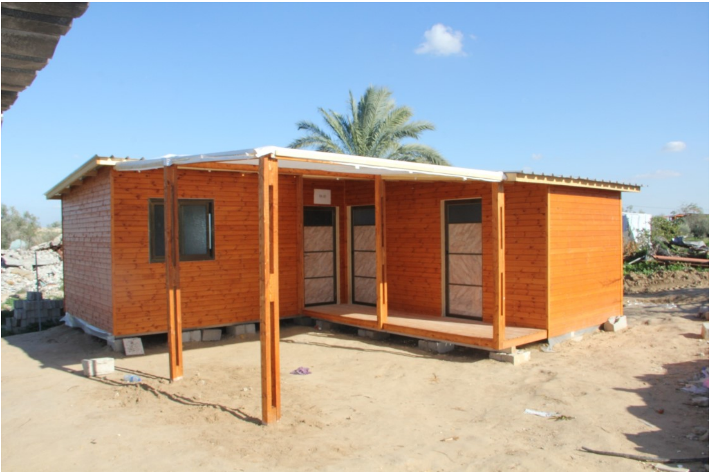
Transitional shelter built with timber, one of the few materials available in the market at the time, 2014.
