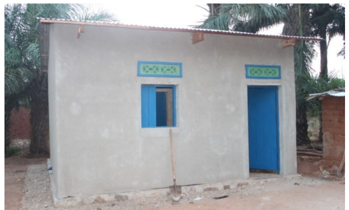
One bedroom, durable shelter with external plaster, 2019.
