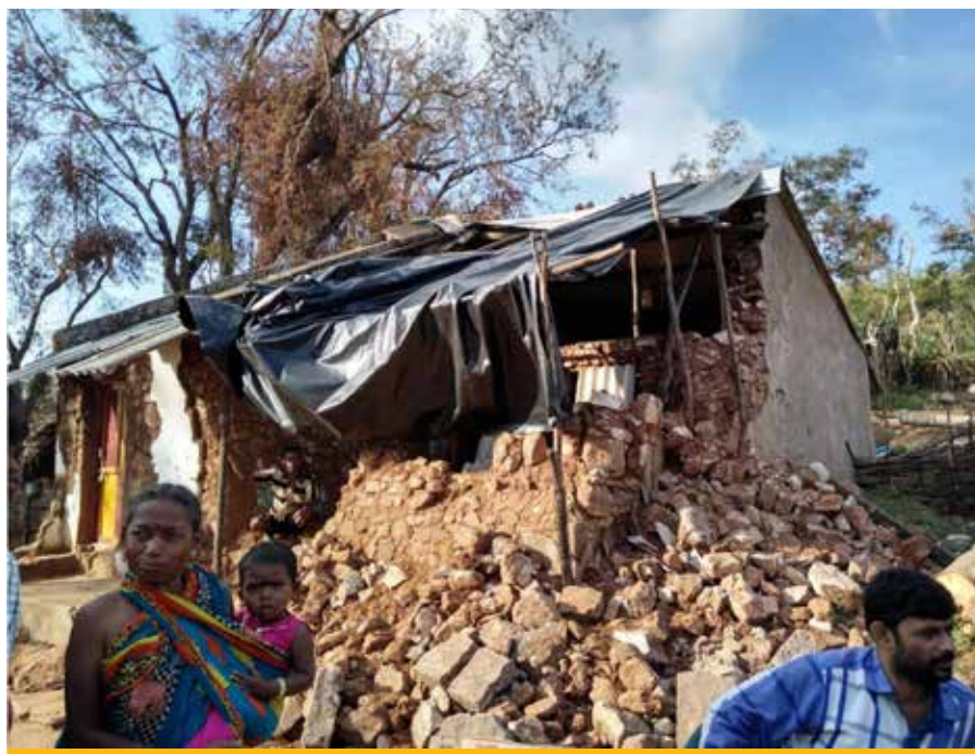
Most houses in the affected areas are made of mud, or a mixture of mud and cement. Photo by Padmakeshari Sahoo/CRS
