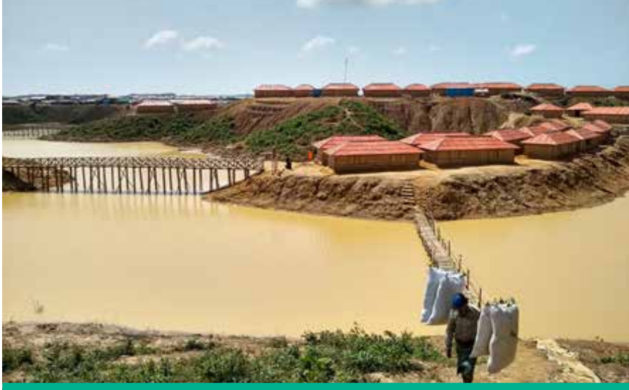
Midterm shelters have been completed in one of the camp extensions. Photo by CRS staff
