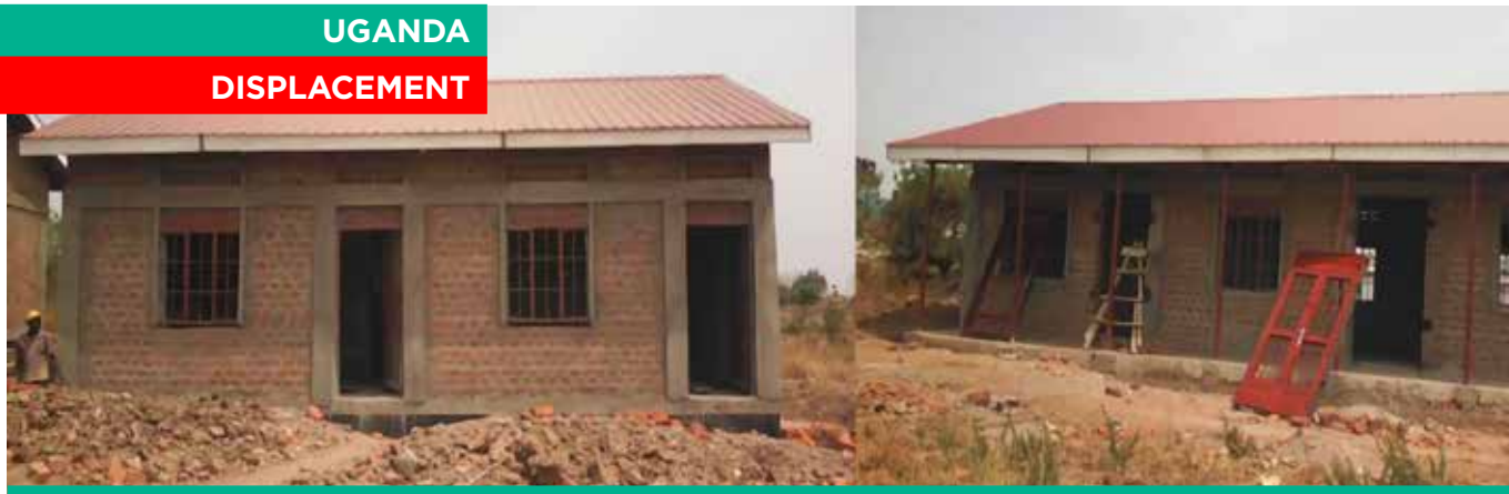
A newly constructed teacher's residence and an administration block at Ariwa Primary School. Photo by CRS staff
