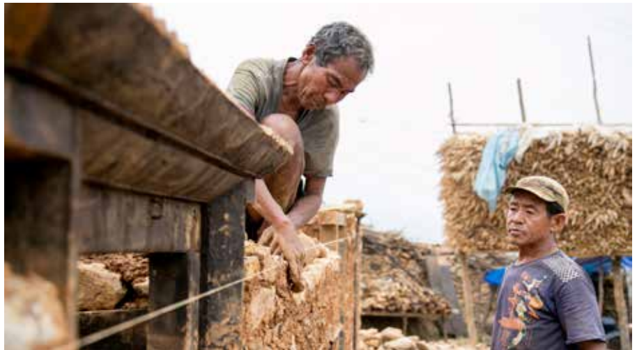
Dal Bahadur Rana Magar constructs an earthquake-resilient home in Gorkha after taking part in a CRS training. Photo by Jen Hardy/CRS
