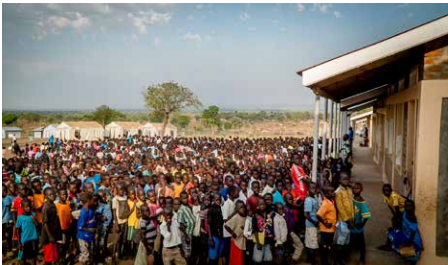
The CRS-built Ayivu Primary School opens new classrooms in the Bidi Bidi Refugee Settlement. Photo by Karin Bridger for CRS
