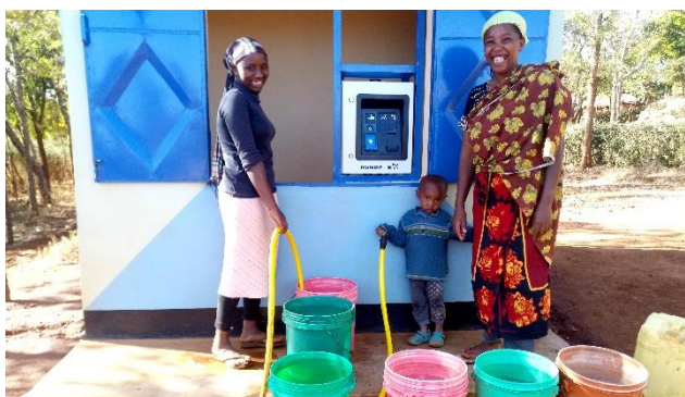
A prepaid water meter in Karatu. The Ministry of Water announced the national adoption of the prepaid water meter on 1 June 2021 [Photo by CRS]
