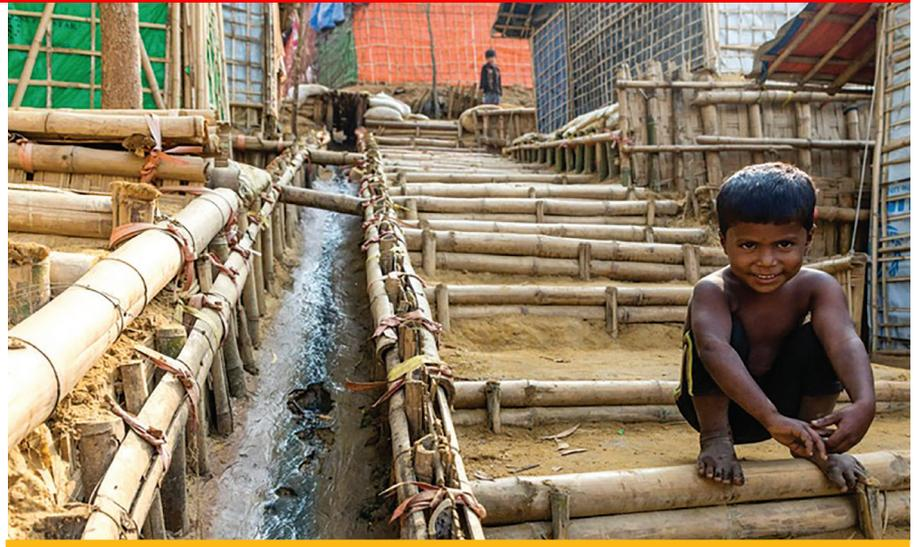
Through a CRS cash-for-work activity, Rohingya refugees used local materials to build structures such as drainage and terraces to mitigate erosion and flooding in the refugee settlement. Photo by Christopher Reichert/CRS
