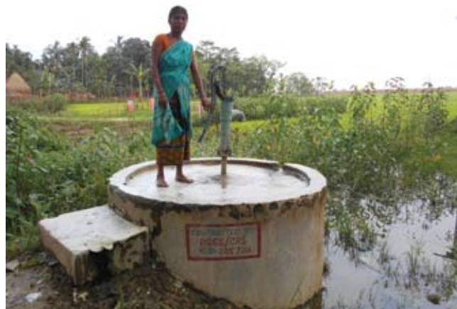
The raised tube wells will give communities potable water during floods for years to come. Photo by Geeta Mazumdar/CRS
