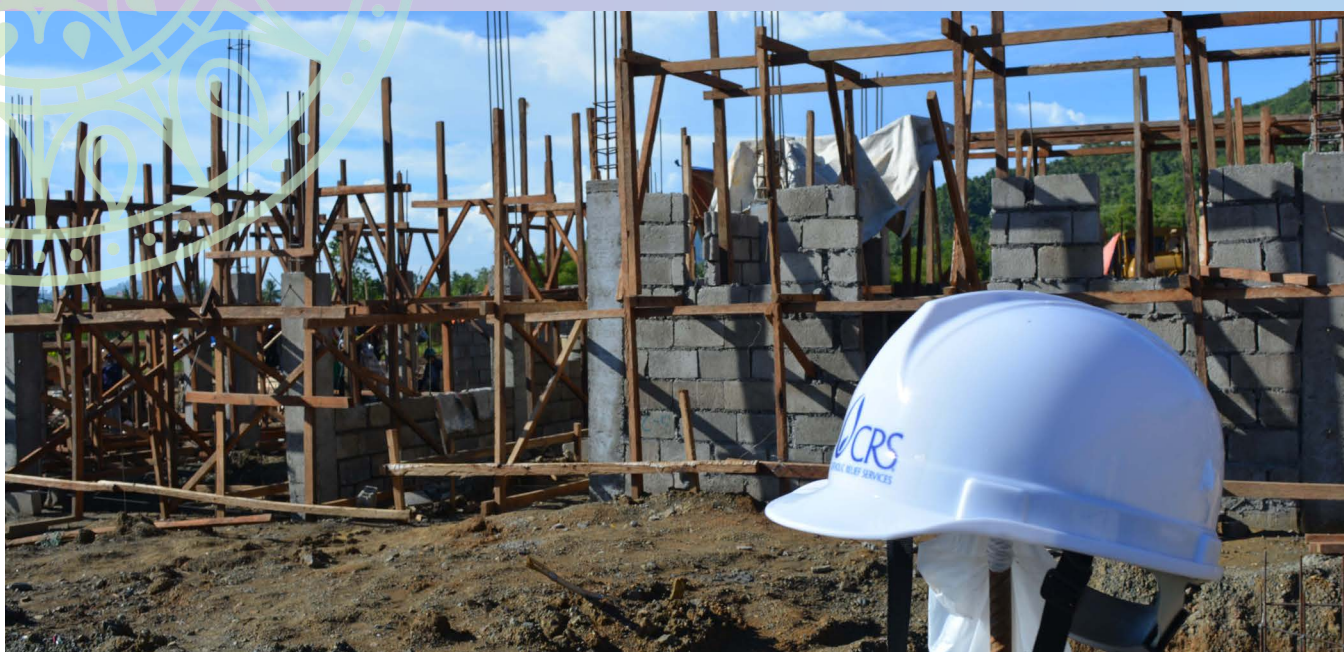
Ongoing construction in Anibong Resettlement Project site in Brgy Bagacay, Tacloban City. Photo by Ma. April dela Cruz/CRS.
