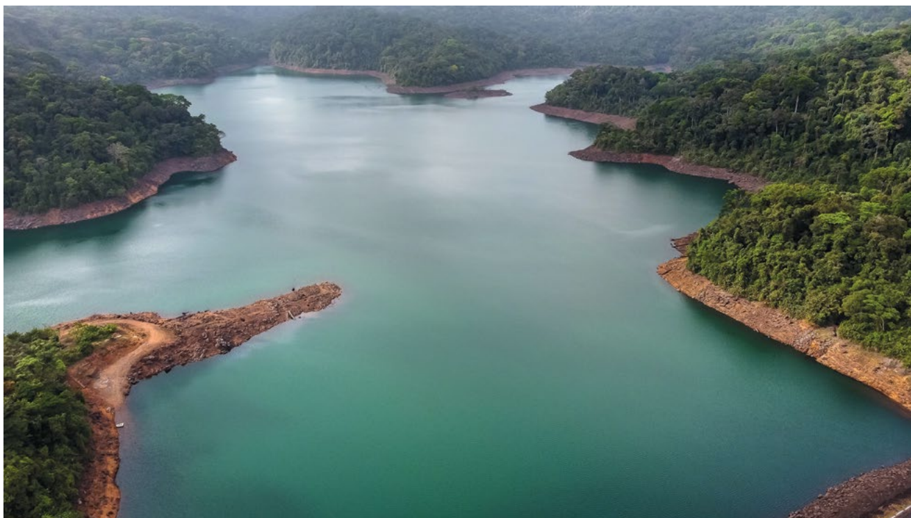
Guma Valley Dam located at Mile 13
