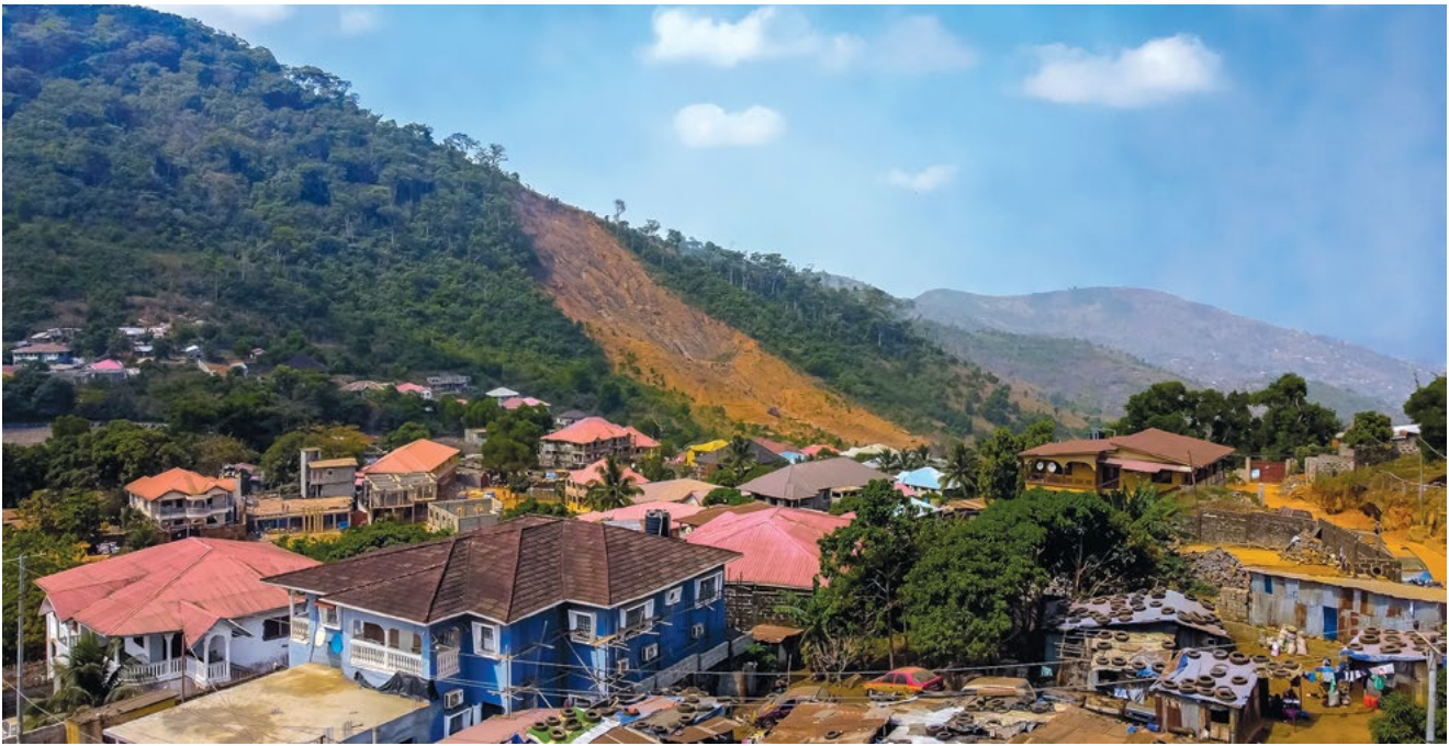
2017 landslide site on Mount Sugarloaf located at Motomeh
