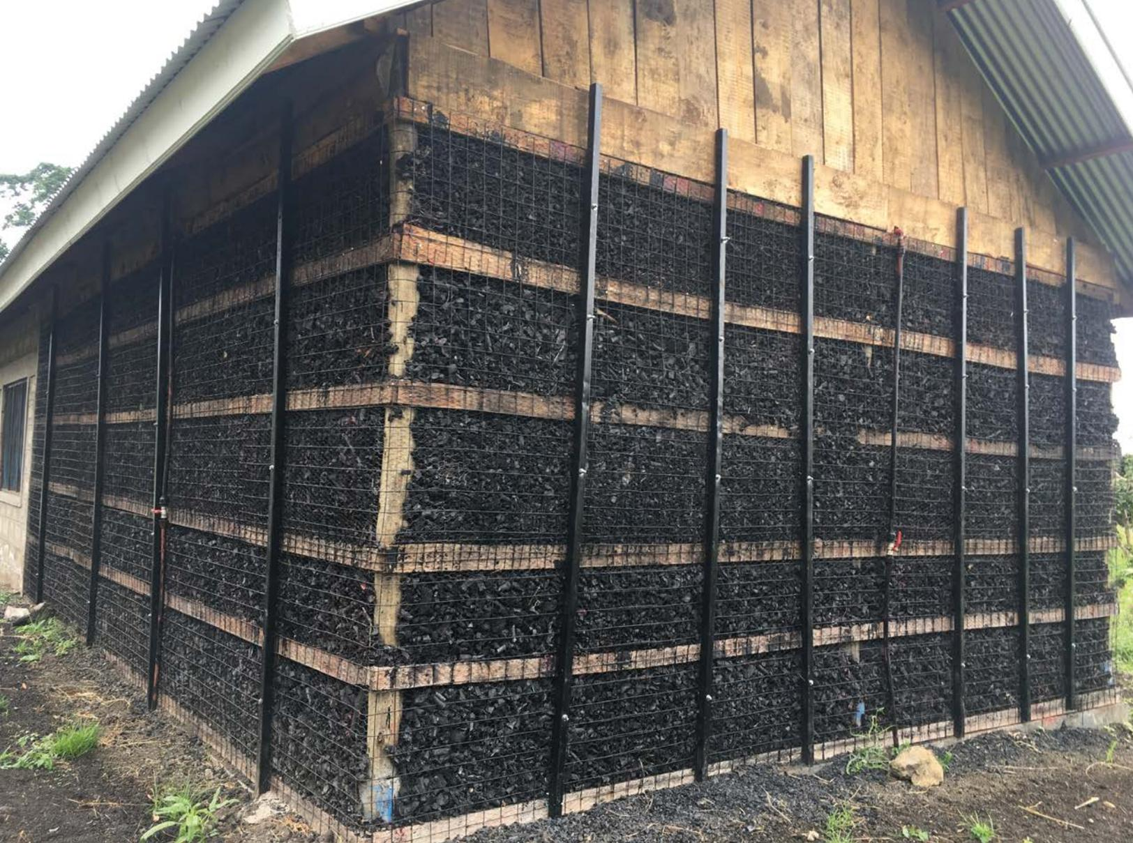
Cold storage room in Tanzania using charcoal-filled siding. The appropriate technology creates conditions for cold storage without the use of fossil fuels.
