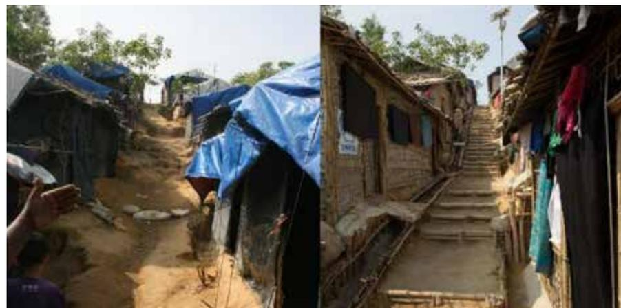
**Before and after:** Through a CRS cash-for-work activity, Rohingya refugees used locally available materials and techniques to build drainage structures and terraces to mitigate erosion and flooding in the refugee settlement. *Photos by Christopher Reichert/CRS*
