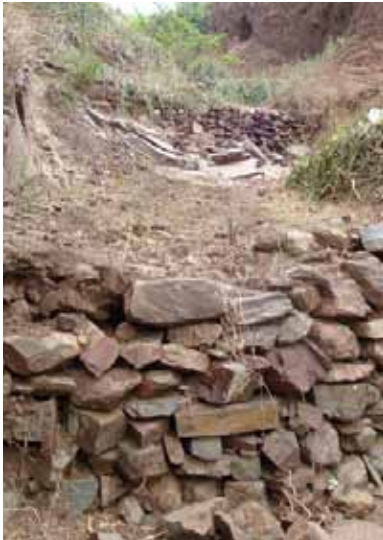
A check dam slows water from flowing down a gully and taking topsoil with it, and it increases water infiltration into the soil. Paul Hebert for CRS.
