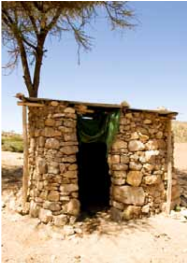
An Arborloo ecological toilet with a rock superstructure, Legedini. Rock is abundant in Legedini and this dry-stack rock superstructure is easily and quickly constructed. Paul Hebert for CRS.
