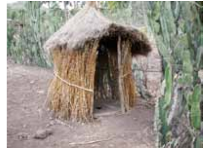
Innovative very low cost "Arborloo" toilet in Harbu. After a year or less of use the slab and superstructure are moved to a new location and a tree seedling is planted on the pit. Tsegahun Tessema for CRS.
