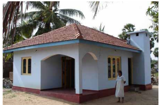
Permanent housing project in Sri Lanka, post-tsunami, 2006 Photo Credit: CRS
