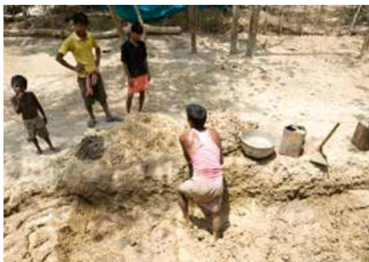
A neighbor helps CRS program participant Purna Chandra Dalai prepare a mud and straw mixture for his new home, built to be flood resistant using techniques and materials taught and provided by CRS. Photo by CRS
