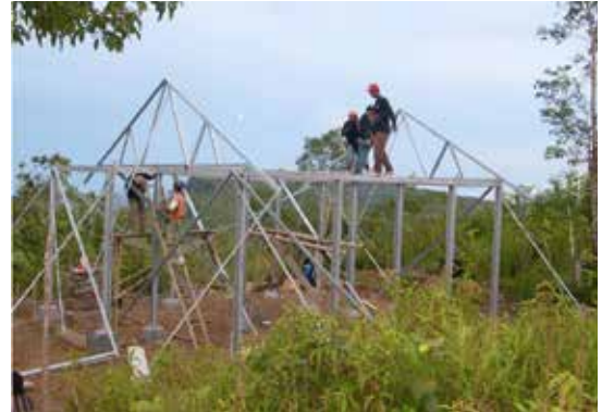
Construction in progress of 45sqm permanent housing in mountain village of Nias Photo Credit: Ariel Sadural for CRS
