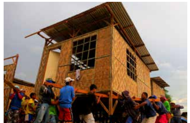
In Philippines shelter response, the transitional shelter was designed to be re-locatable and demountable Photo Credit: Charisse Mae Q. Borja for CRS
