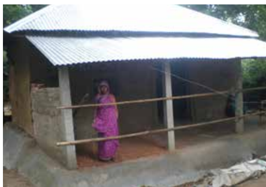
Completed flood-resistant shelter. Photo by CRS
