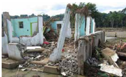
House destroyed by flash floods Photo Credit: Charisse Mae Borja for CRS
