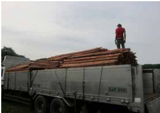
Coconut timber delivery to construction site Photo Credit: Chin Lovi for CRS
