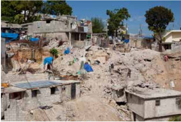
Destroyed urban houses after earthquake in Port-au-Prince, Haiti, 2010, Photo Credit: Benjamin Depp for CRS
