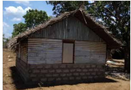
Completed transitional shelter Photo Credit: CRST
