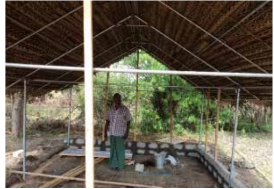
Construction transitional shelter Photo Credit: CRS
