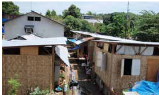
Transitional shelter on site in Cagayan de Oro Photo Credit: Seki Hirano for CRS
