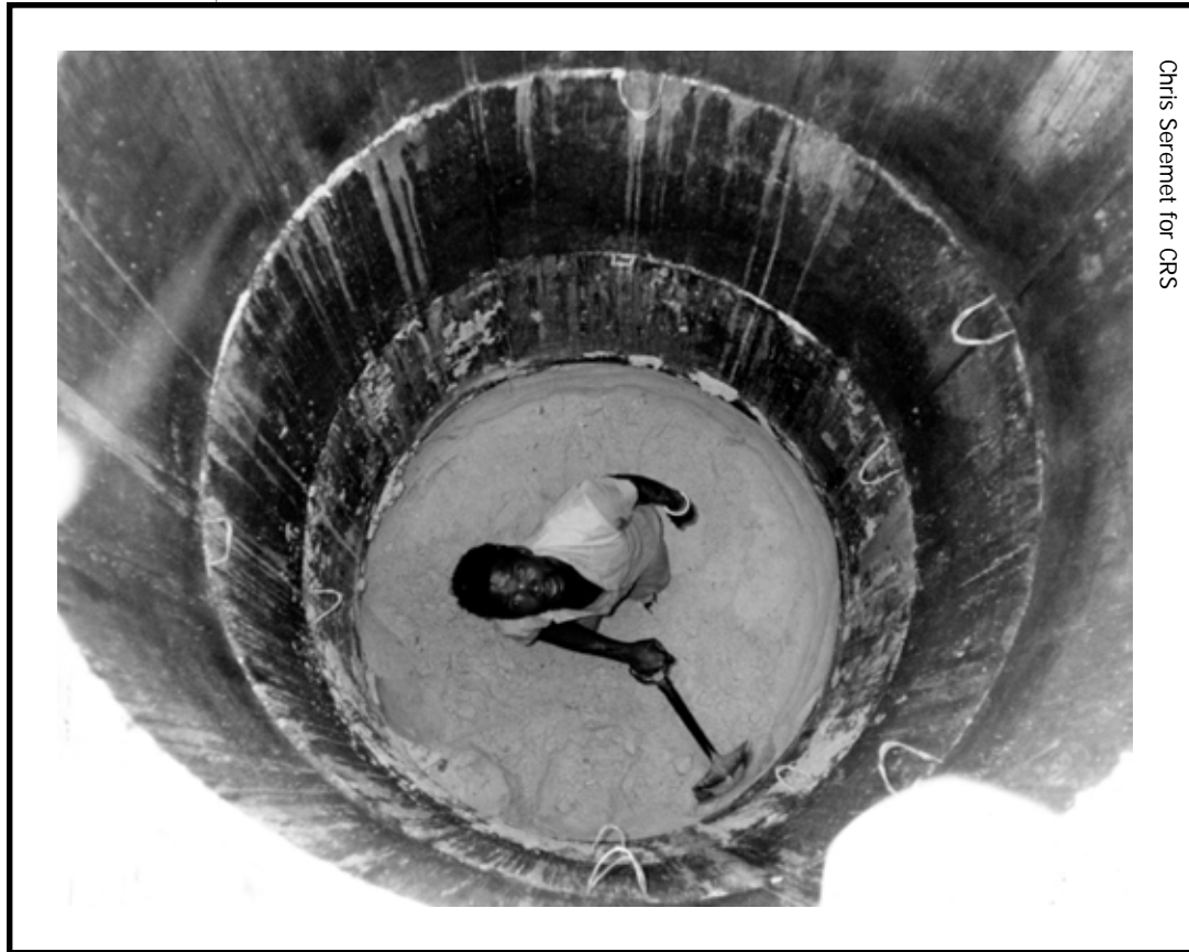
A man digging a well in sandy soil in Namibia.
