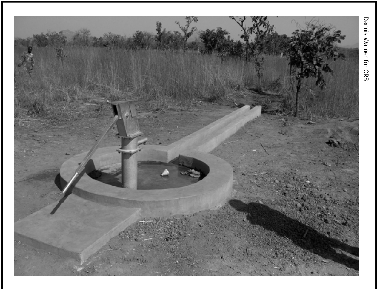
A bored well installed with a handpump, concrete apron, and concrete spillway in Sudan.
