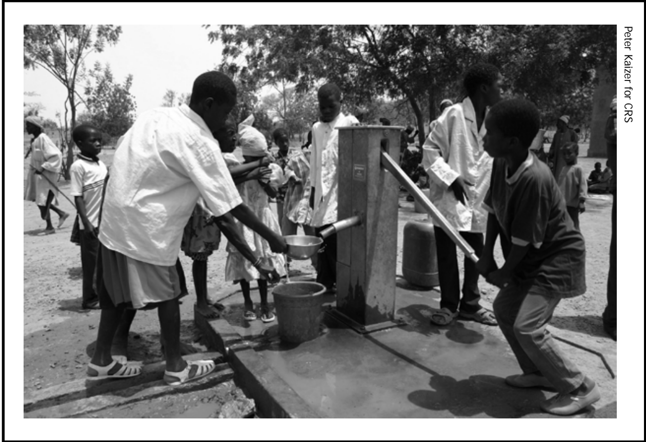
A handpump used to supply groundwater to a school in Burkina Faso.
