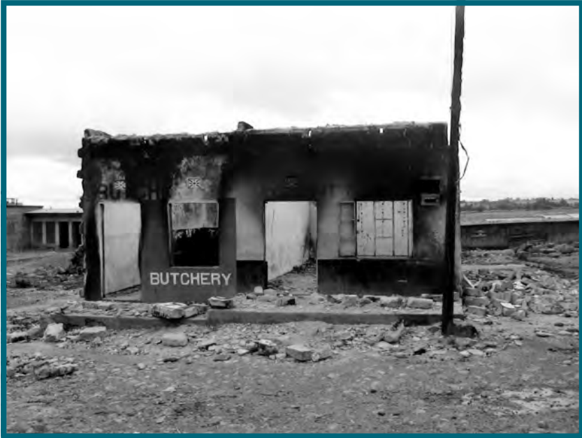
An example of the damage inflicted by the 2008 post-election violence in Burnt Forest.
