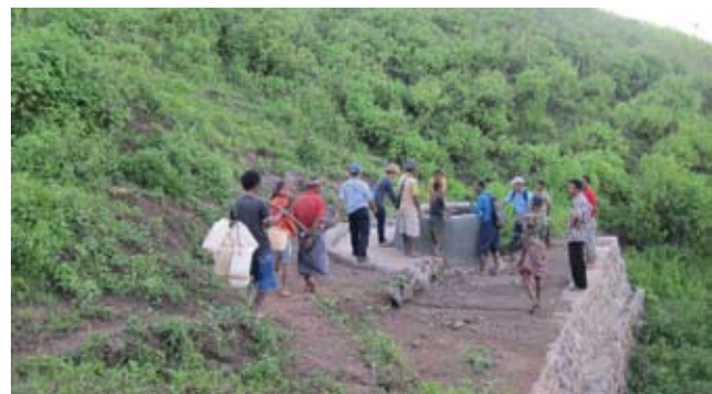
A slope during and after landslide protection work. Photo by CRS staff
