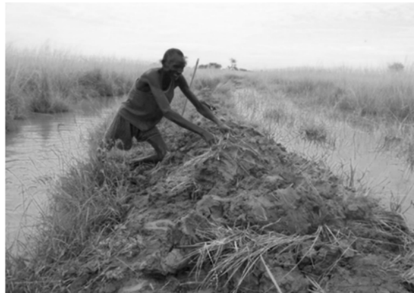
Building a dike through Food for Work in South Sudan
