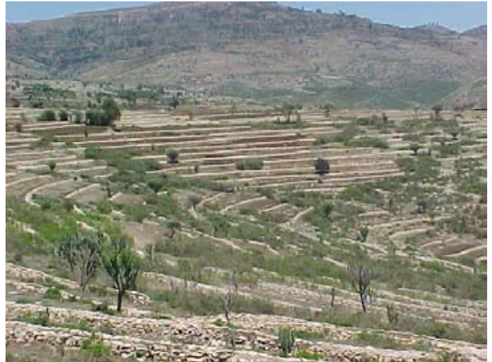
Hillside terracing helps Ethiopian communities to replenish natural water sources for significantly improved quality of life. Photo by Zemed Abebe/HCS
